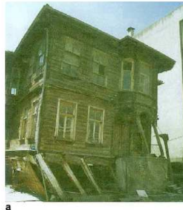
Fig. 13. Heavily damaged traditional wooden buildings due to soft story. (a) Large laterally displaced traditional building [26]. (b) Laterally displaced traditional building [20].
