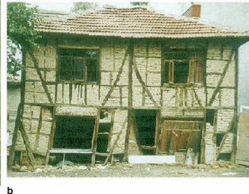
Fig. 13. Heavily damaged traditional wooden buildings due to soft story. (a) Large laterally displaced traditional building [26]. (b) Laterally displaced traditional building [20].
