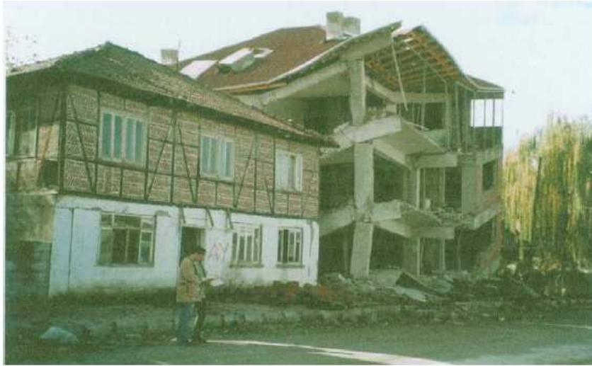
Fig. 1. View of traditional and reinforced concrete buildings after the 1999 Duzce earthquake.
