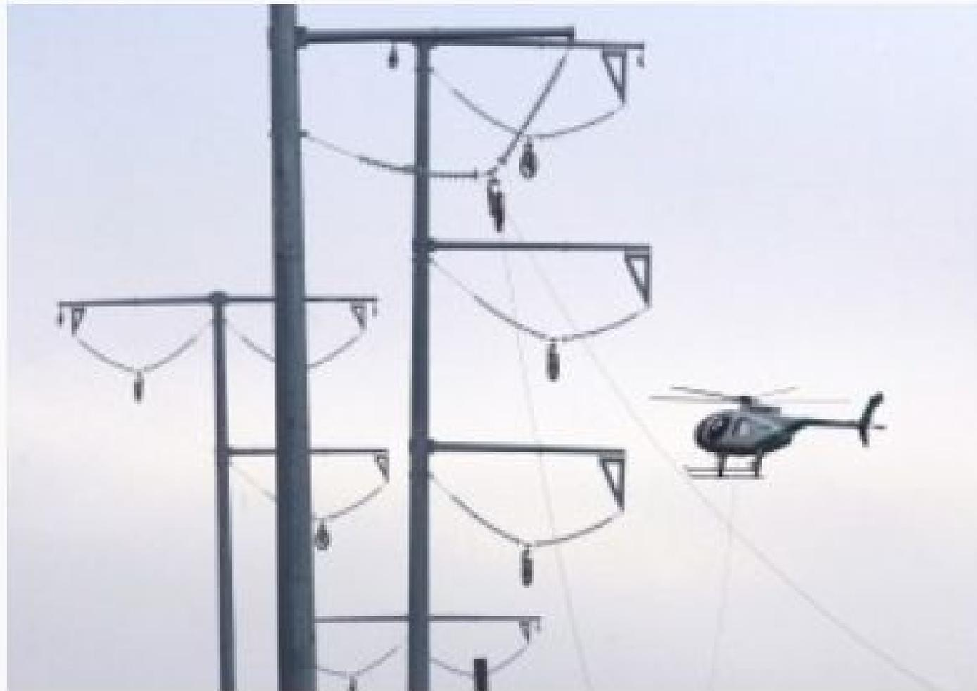
*A helicopter starts the process of stringing a high-voltage transmission line*
